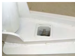
3/8" bolt inside anchor sleeve
